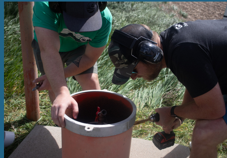
Lower Platte South NRD staff install telemetry units on wells, which will automatically collect and transmit data from the remote source.
