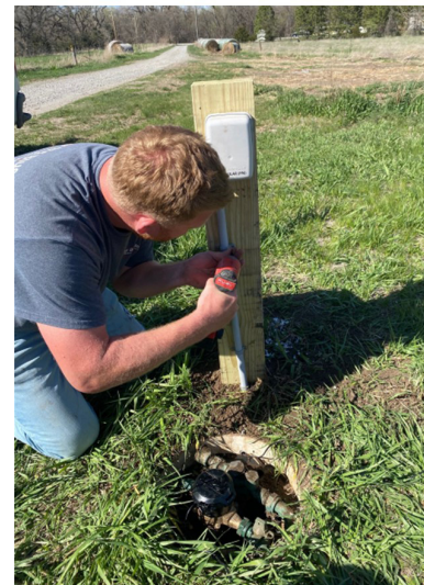
Lower Big Blue NRD Water Resources Specialist Ryan Thomas completes installation of a new water meter and cellular meter interface unit on the District's Beatrice West Rural Water Project.
