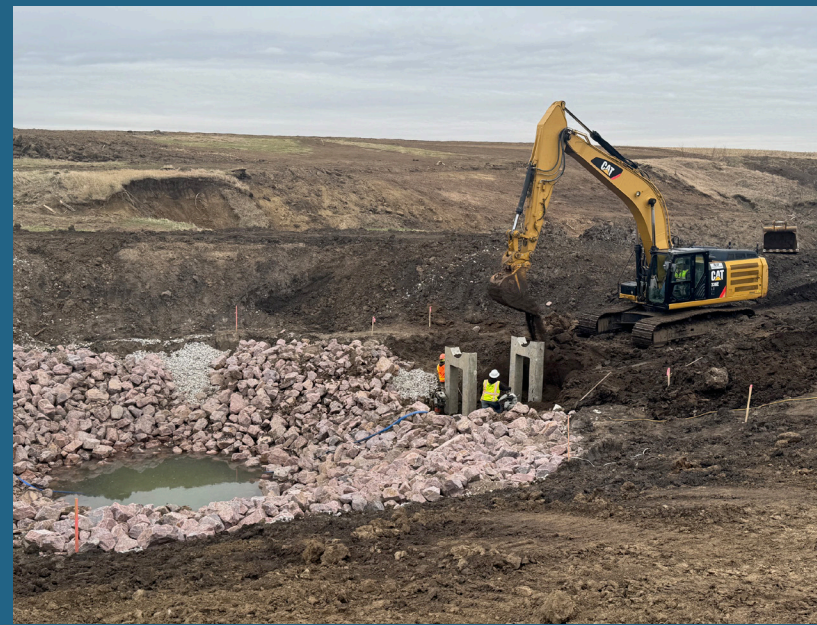
The plunge pool spillway outlet is placed for site 27 of the Wahoo Creek Watershed dams. This is one of three dams currently under construction in the Lower Platte North NRD with completion slated for fall of 2026.
