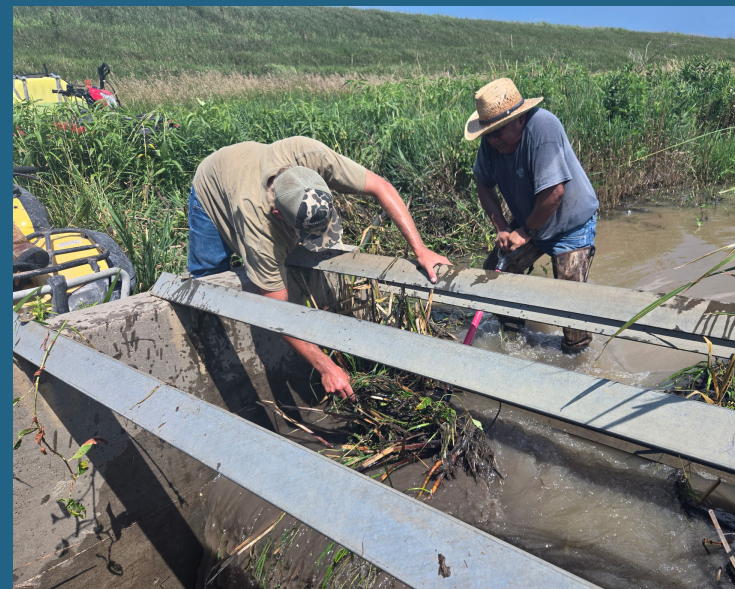
Nemaha NRD Field Technician Tomas Chalé Aké and seasonal staff remove debris from a riser on one of the district's watershed dams during routine maintenance.
