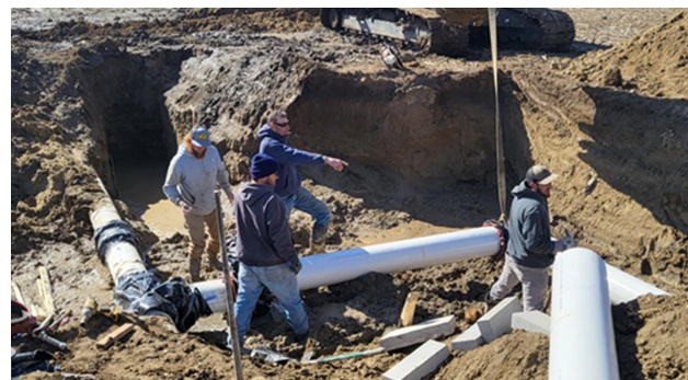
Lewis & Clark NRD installs new water distribution lines during Phase I of the Cedar-Knox Rural Water Project.
