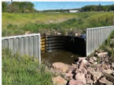
Toe wall structure. Standing in drainage area to Shell Creek, looking up towards meadow.
