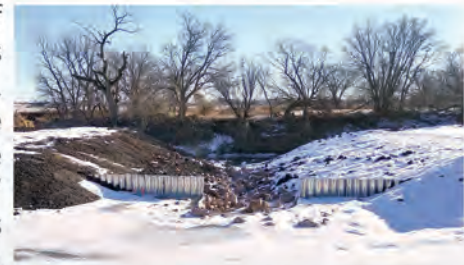
Toe wall structure nearly completed looking towards the drainage area into Shell Creek.
