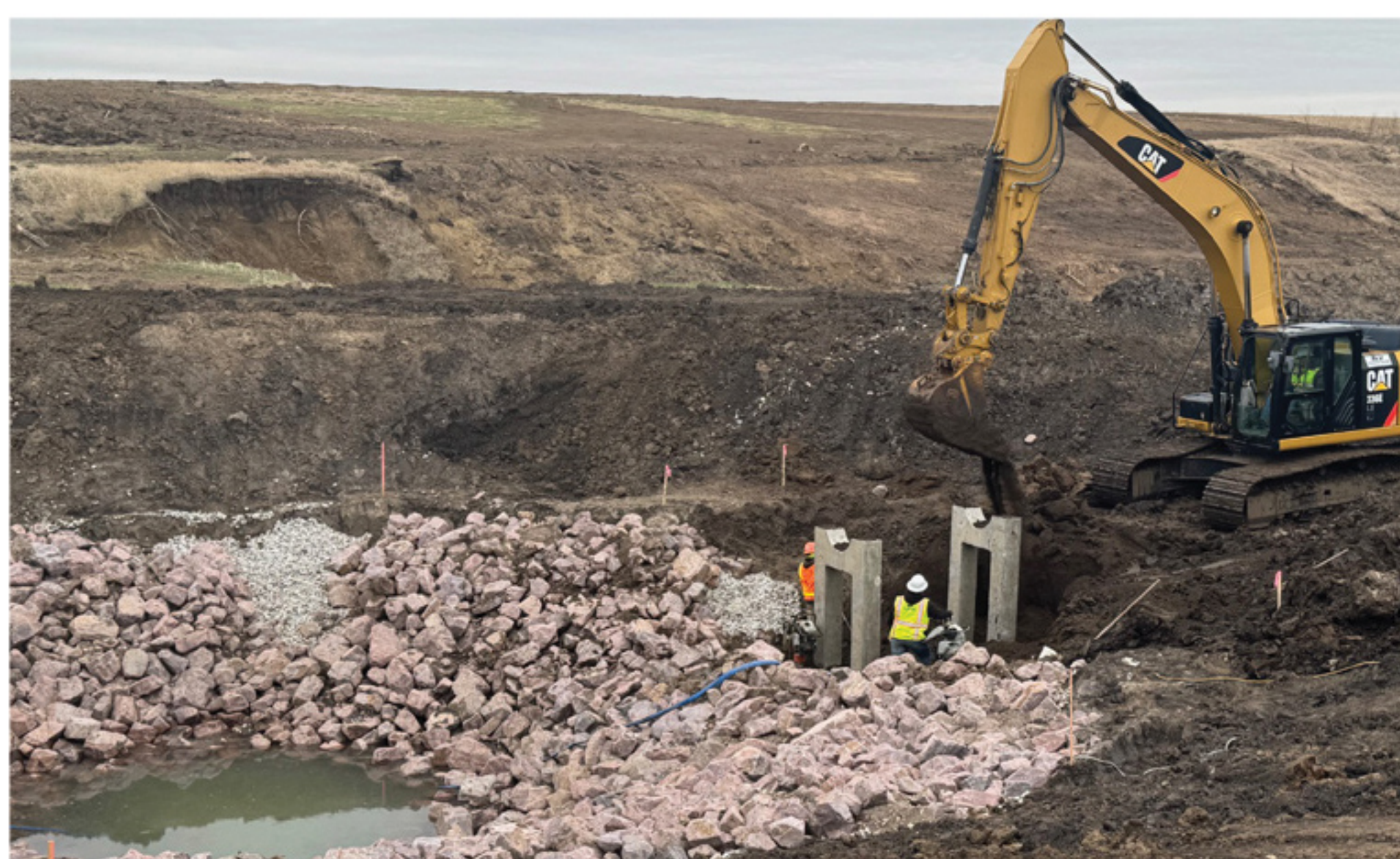
Thompson Construction, Inc. works on the plunge pool spillway outlet for site 27.
