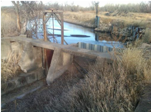
(Above) Diversion gates from the Platte River to the Six Mile Canal. (Right) Map of the Six Mile Canal.
