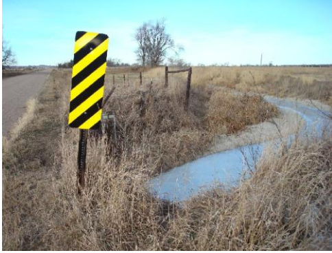
(Above) The removal of the canal protects lives, saves the county dollars and improves roads through reduced maintenance costs while removing bridges and other hazards to drivers within the road right-of-way.
