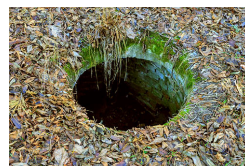
Old wells such as this pose a threat to your health, safety and the environment.
