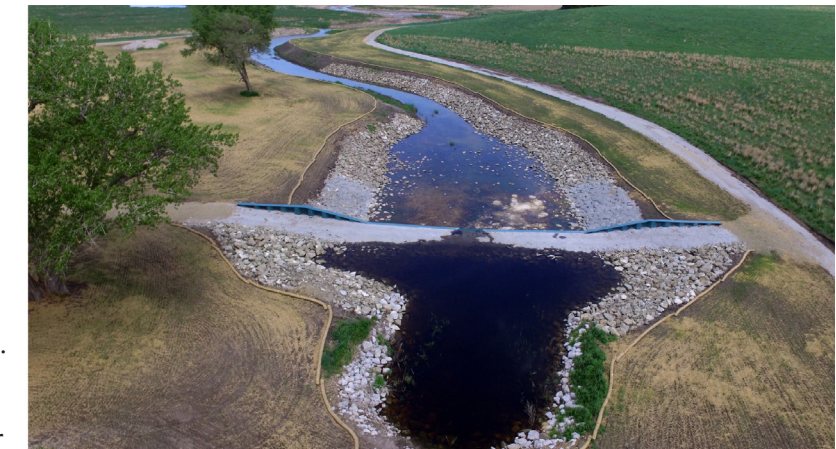
New sheet pile drop structure with grouted low water crossing, Silver Creek and Schaubsville Road.
