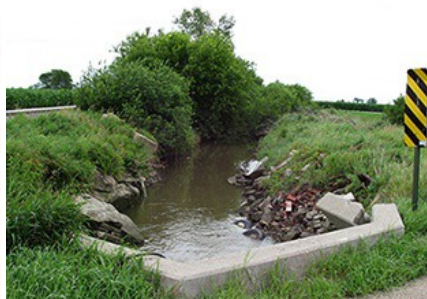
(2012): Channel overgrown with trees and channel in disrepair.
