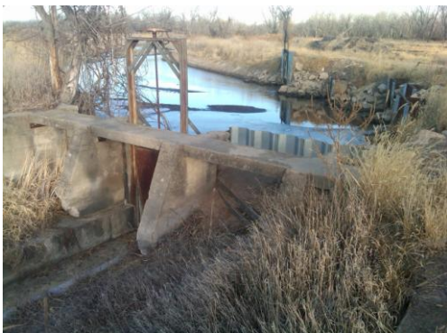
(Above): Diversion gates from the Platte River to the Six Mile Canal.
