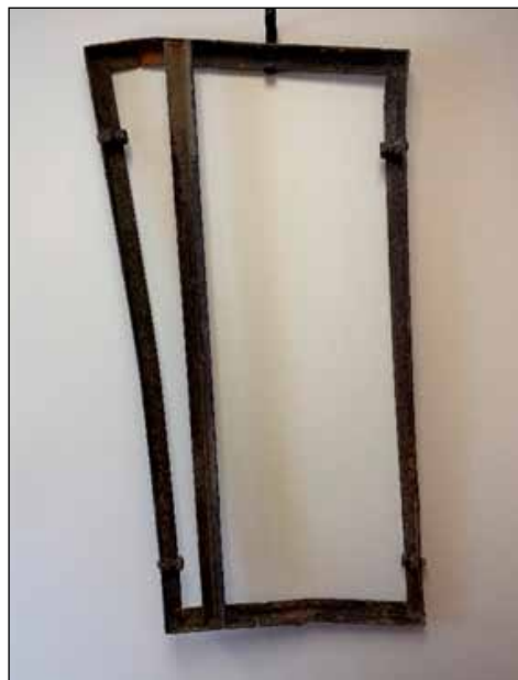
The metal grate that caused the blockage.
