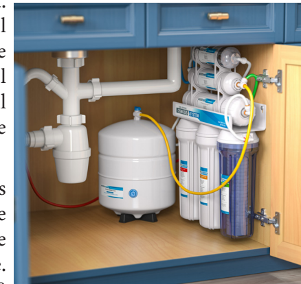
A reverse osmosis system installed under a kitchen sink.
