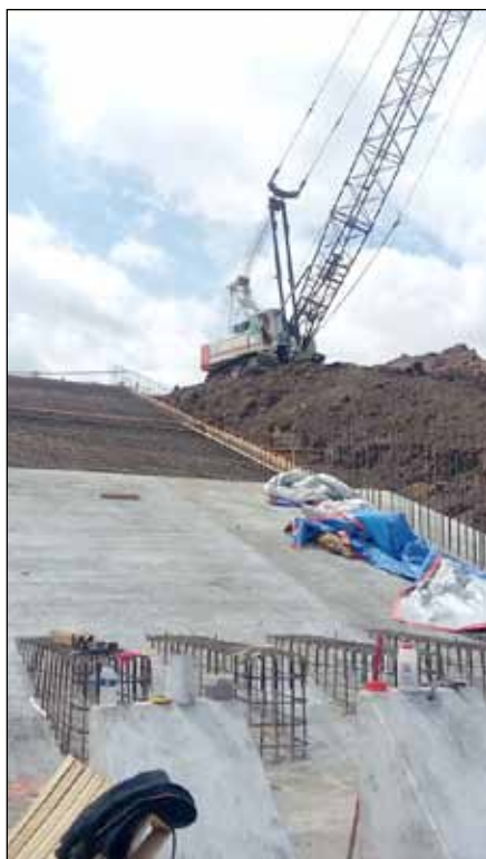
Construction continues on the concrete work at UBN 25-C.
