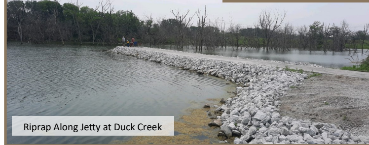
Placing Riprap at Duck Creek
