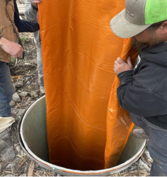
Installing the UV Liner
