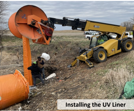
Installing the UV Liner
