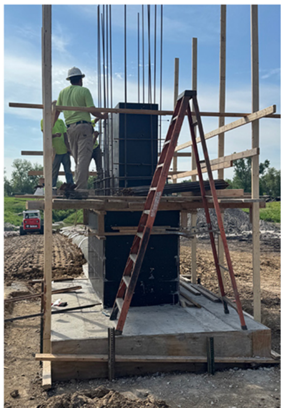
The riser inlet under construction at site 27.
