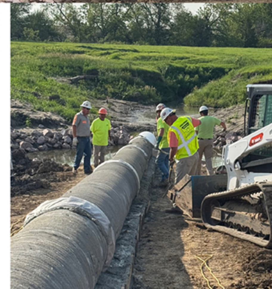
Workers grouting the 24" concrete pipe spillway.
