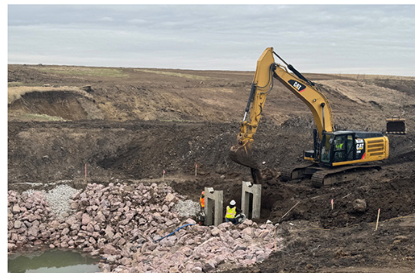
The plunge pool spillway outlet for site 27.
