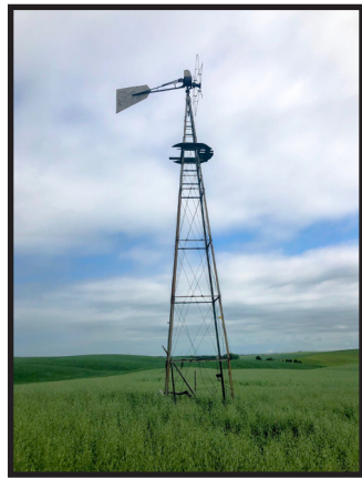
Well Prior to Decommissioning
