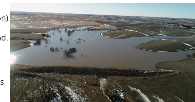
PCLU 4, one of four dams in Prairie Creek Watershed, located 15 miles west of Grand Island. The deepest area held 12 to 14 feet of floodwater near the dam.
