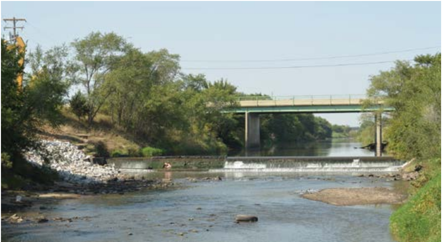
This weir on Oak Creek has required almost no maintenance since it was built in the 1940s. The First Street Bridge is also pictured.
