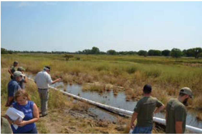
The NRD staff is briefed on the salt water irrigation system installed this summer at Marsh Wren Saline Wetland. See LPSNRD.org for more photos.
