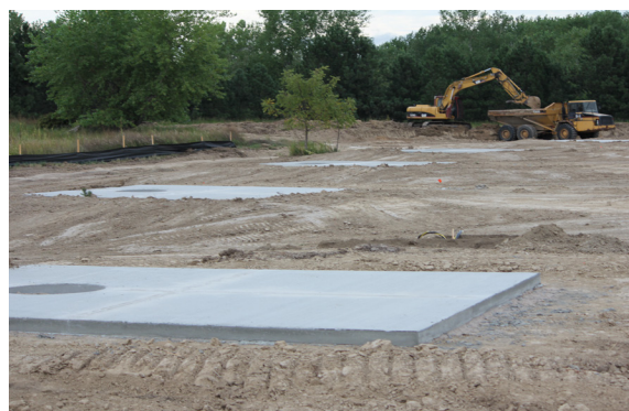
Davis Creek camper pads have been poured.
