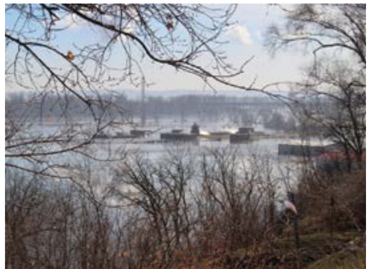
Plattsmouth’s wastewater treatment plant lost power due to March flooding. The city was still assessing flood damage in May.
