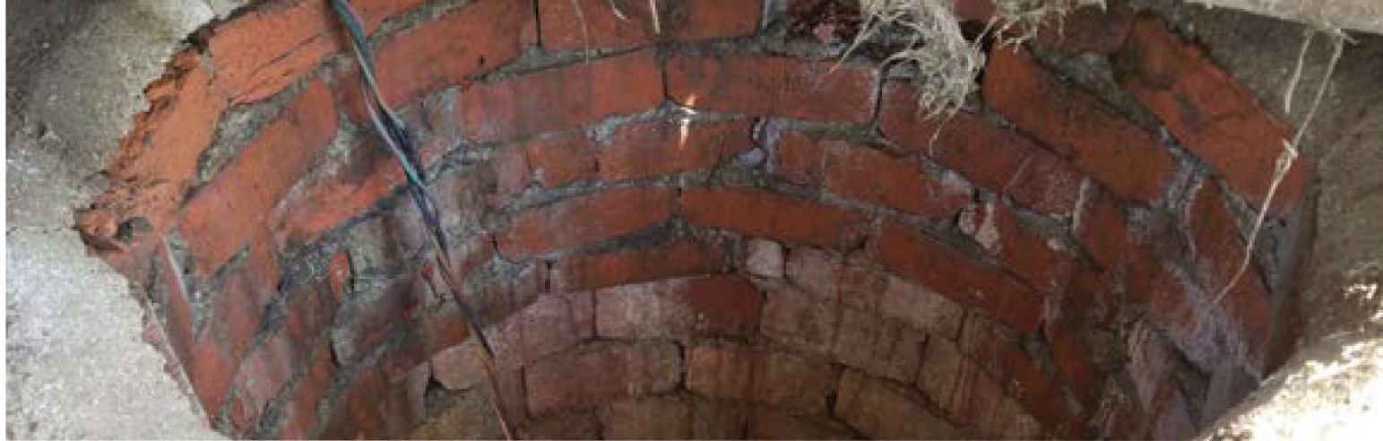
This hand-dug well (30 inches in diameter and 33 feet deep), on property owned by Mark Nutzman, in Otoe County, was decommissioned last November.
