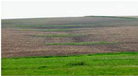
Looking upslope at a series of parallel water and sediment control basins built across a small watercourse on a cropped hillside. Photo courtesy MN NRCS.
